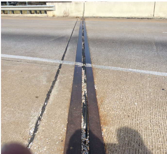
PHOTO 1 Description Dirt and debris in expansion joint assemblies.
