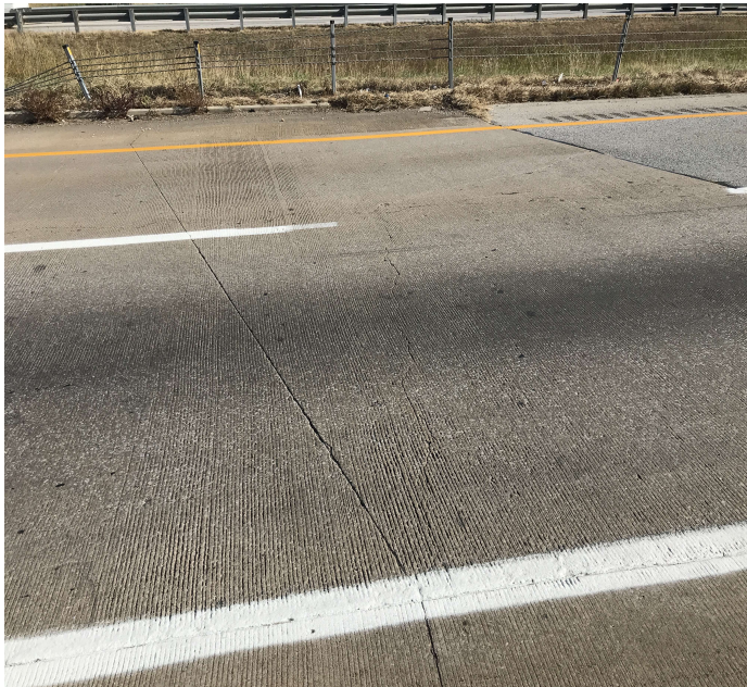
PHOTO 1 Description Longitudinal and transverse cracking in south approach slab
