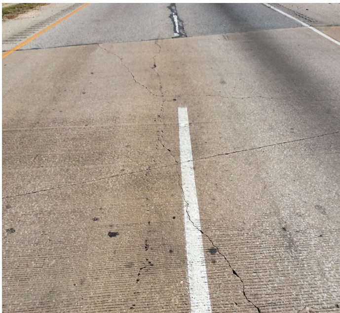
PHOTO 3 Description South approach slab-Longitudinal cracking.
