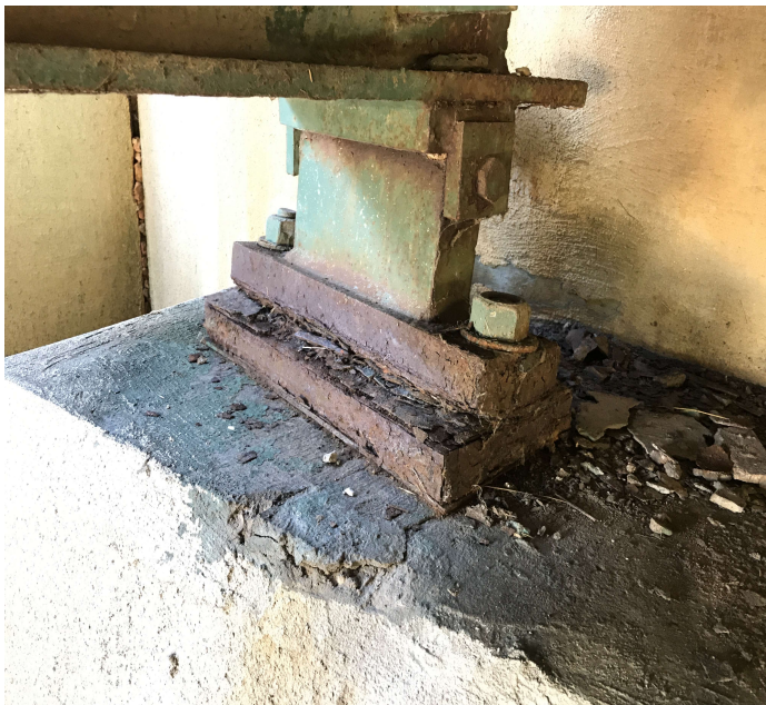
PHOTO 1 Description Bearings #6 abutment #1 pack rust.
