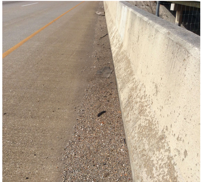
PHOTO 2 Description Dirt and debris in right gutter.
