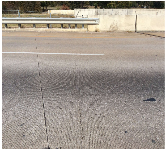
PHOTO 2 Description North approach slab-Transverse cracking.
