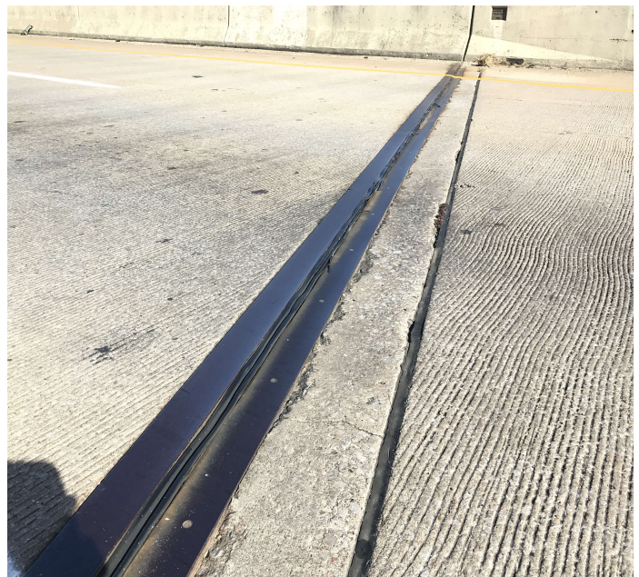
PHOTO 2 Description Abutment #1 expansion joint tearing and cracking
