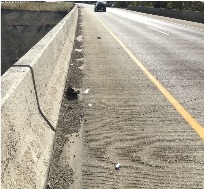
PHOTO 1 Description Right gutterline dirt and debris accumulation
