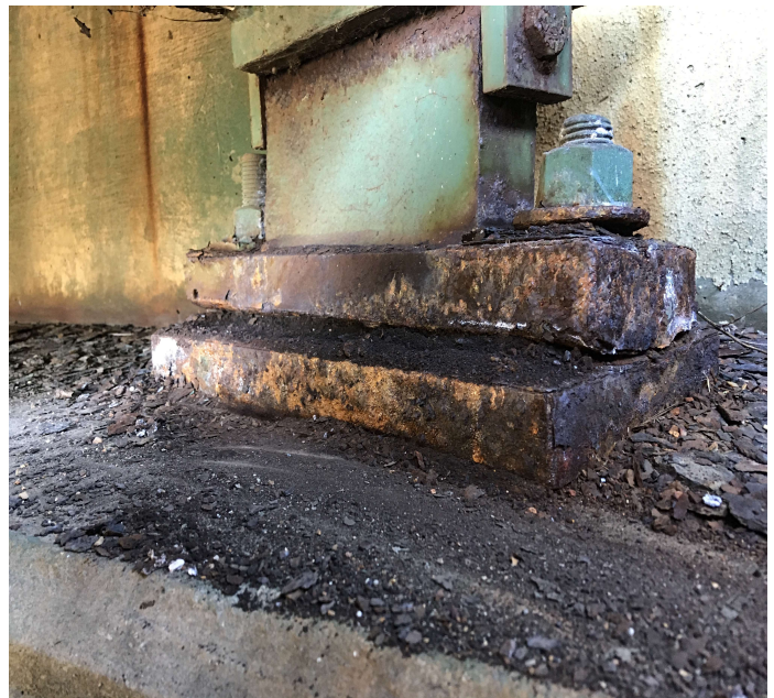
PHOTO 2 Description Abutment #2 bearing #6 flaking rust.
