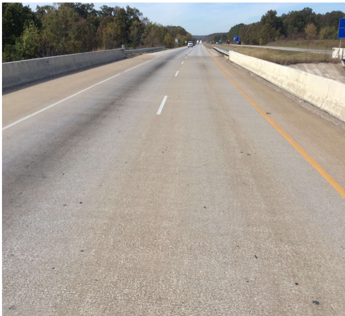
PHOTO 4 Description Deck has sealable cracking in all spans.
