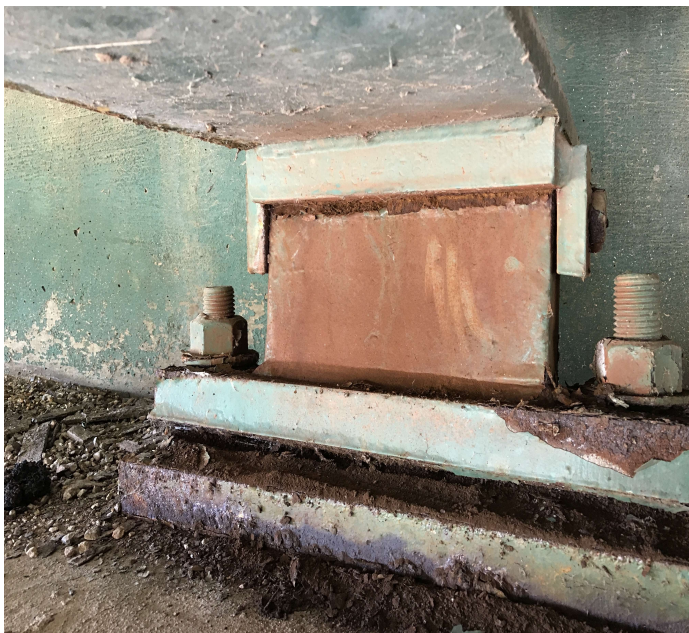
PHOTO 3 Description Abutment #2 bearing #2 fretting between rocker and sole plate.
