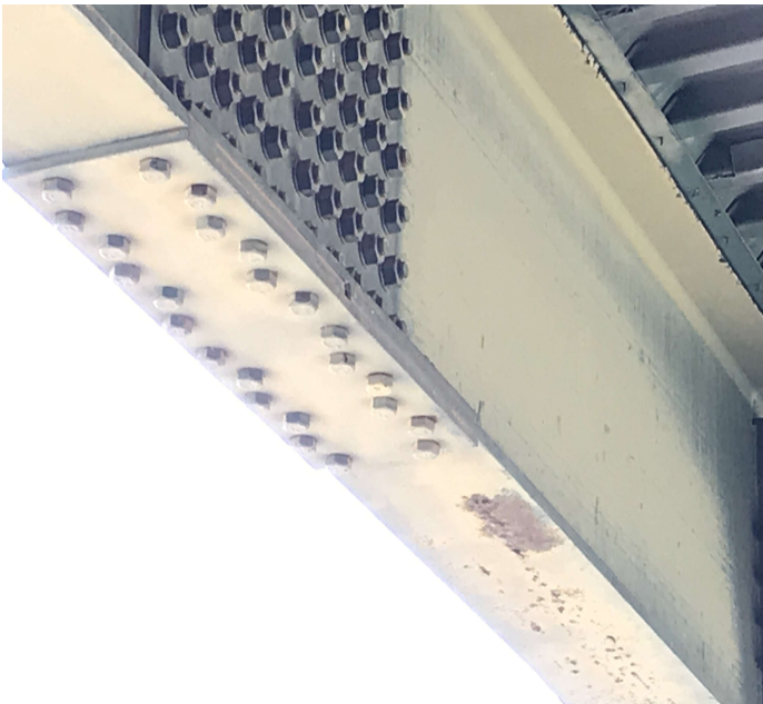
PHOTO 3 Description Span #3, Girders #6 have one loose bolt in the bottom flange splice plate connection.
